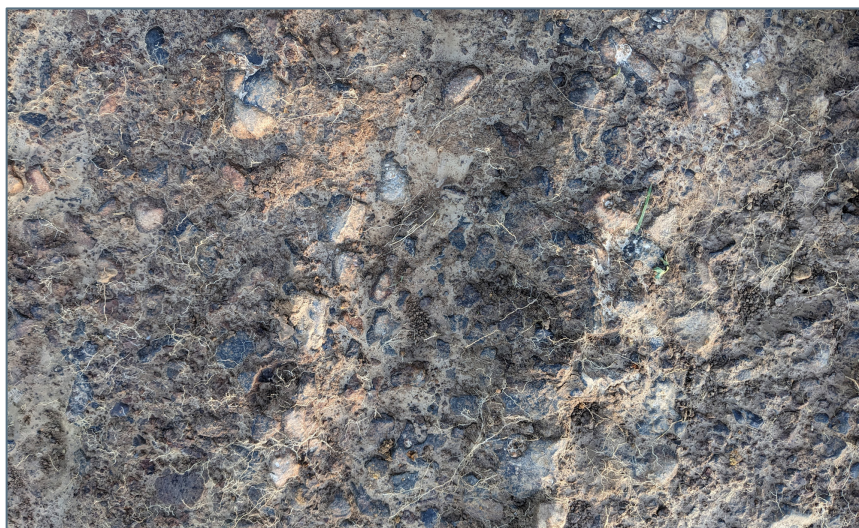
Figure 1: Rochester Roman road at Icklesham, showing wheel rut in crushed slag surface
